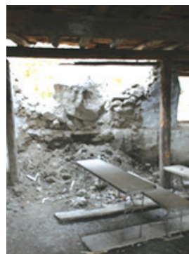
A large stone fell on a school in Shreenagar in August 2009 – No children were in the classroom.
